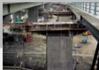
and two abutments were built to support the new deck. Road closure was limited to a weekend – eight hours for the slide, 24 hours to allow bearing grout to set and the remainder for asphaltting and traffic re-routing. The merge slide was downhill on a 2.85 % slope. Balance between pushing and pulling forces gave a controlled pulling force of up to 5,700 kN. Pulling was incremental, governed by the jack stroke of 600 mm, enabling a rate of travel of up to 1.8 m an hour.
